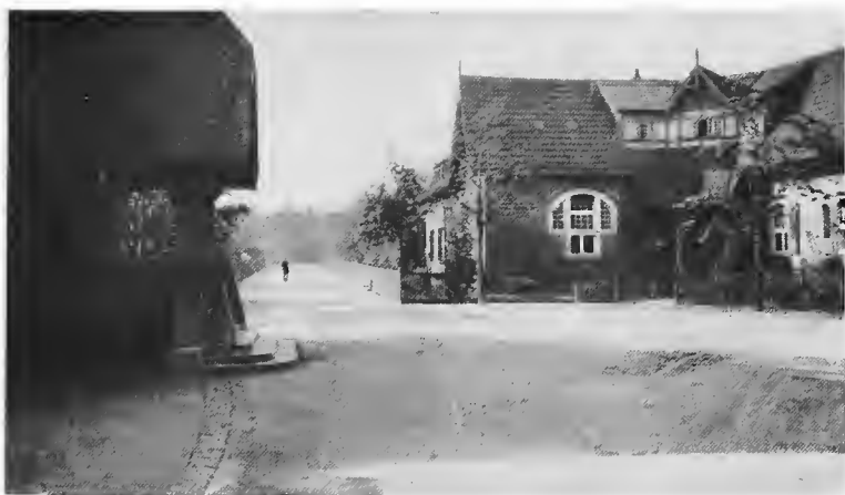
ATTRACTIVE AND INEXPENSIVE STREETS OF THE KRUPP VILLAGES, NEAR ESSEN, GERMANY
