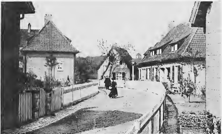
ATTRACTIVE AND INEXPENSIVE STREETS OF THE KRUPP VILLAGES, NEAR ESSEN, GERMANY
